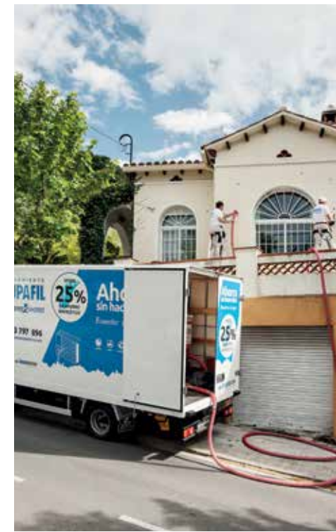
SUPAFIL being installed at a home in Spain through the outside, meaning minimum disturbance to the homeowners.
